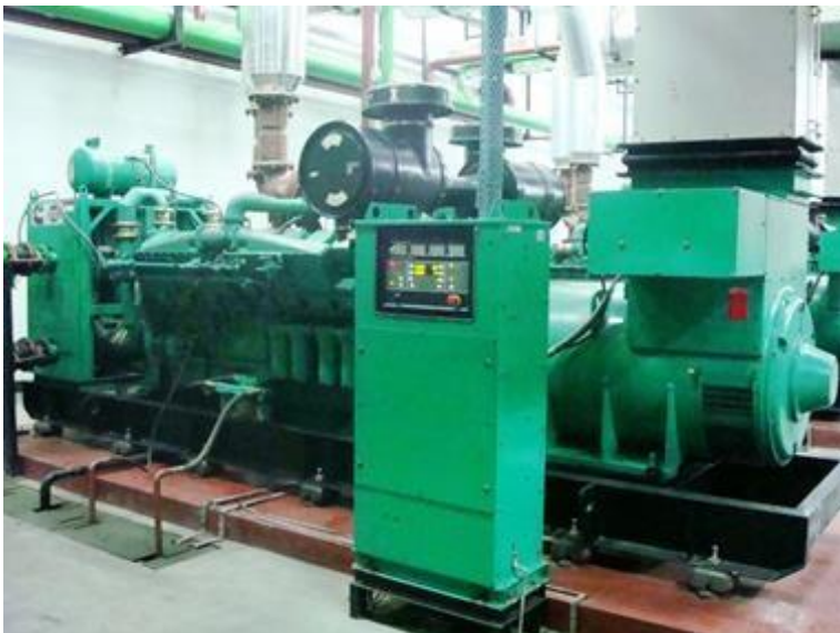
PCC Panel near DG
